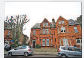
20A Old Park Avenue, Clapham South, SW12
